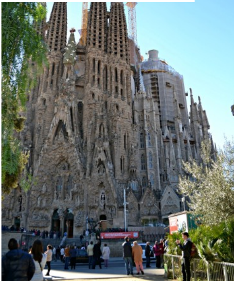
Work continues on Gaudi's La Sagrada Familia
